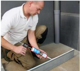
**3** If applying to a stud wall of Marmox board, run a bead of Marmox Acrylic Sealant along the edge of the Marmox pipe boxing.
