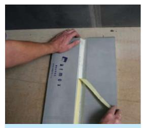
1 Cut to correct length. They come in 1.25m lengths as standard and cut be stacked on top of each other to create height. Remove the tape.
