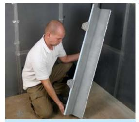
**5** This example shows being fitted in the corner again a stud wall and solid wall. Be sure to mark against the wall and drill out the hole positions.
