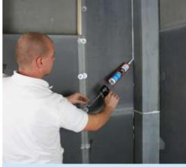
**8** You can seal the edges with Marmox Acrylic Sealant. The Marmox pipe boxing is now ready to be plastered or tiled.
