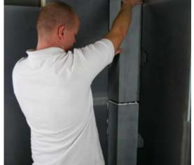
7 Add Marmox Acrylic Sealant / Marmox Wall Brackets to the next piece of Marmox pipe boxing and push firmly into place. Add screws.
