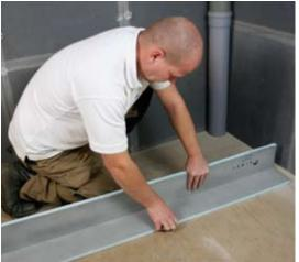
**2** If necessary for extra waterproofing run a bead of Marmox Acrylic Sealant along the fold. Then fold in half to create a 90° angle.
