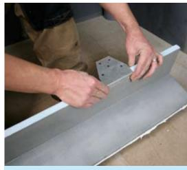
4 If the Marmox pipe boxing is being used against a solid wall then it is recommended to use Marmox Wall Brackets. Use 2 per side of a 1.25m length.
