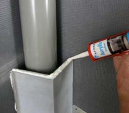
**6** Place the Marmox pipe boxing in place and push firmly. Add screw fixings. Run a bead of Marmox Acrylic Sealant around the top.
